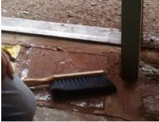
Photo 92 - Access Hatch under Entrance Flooring (with door sill installed)
