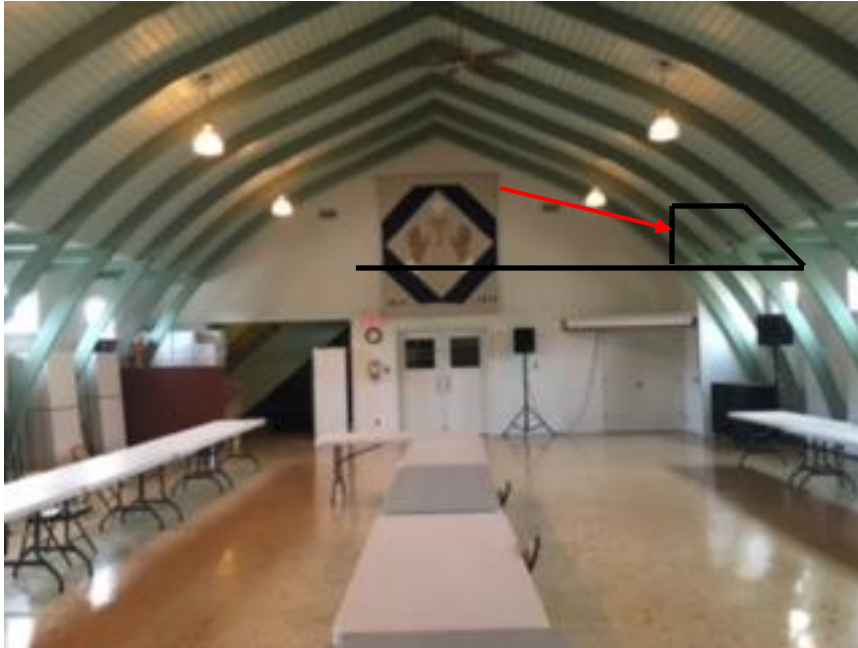
Photo 46 - Location of "Small Storage Room" Over Chair Storage Room
