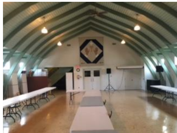
Photo 5 - 2018 View of Parish Hall South Wall (Original Entrance) (south)
