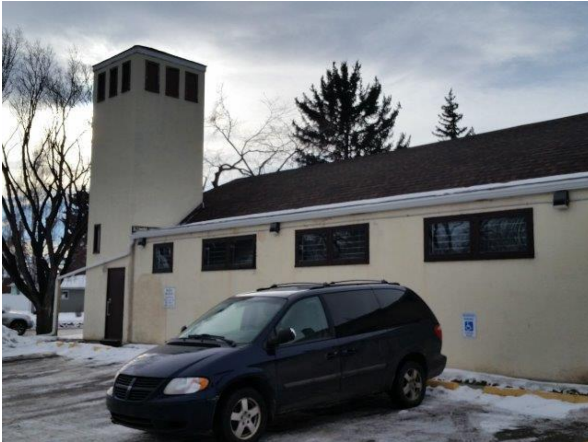
Photo 6 - East Exterior Side of Parish Hall ~2018
