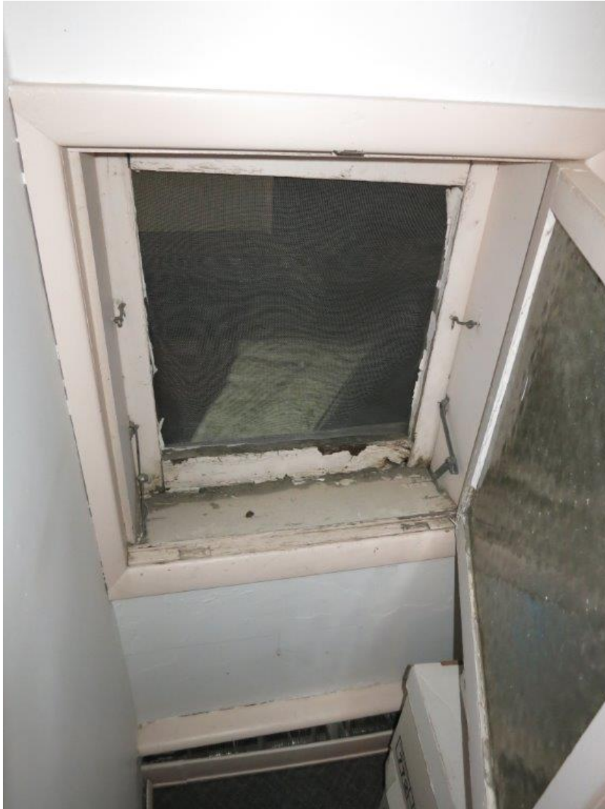
Photo 76 - Upper Office Original Window
