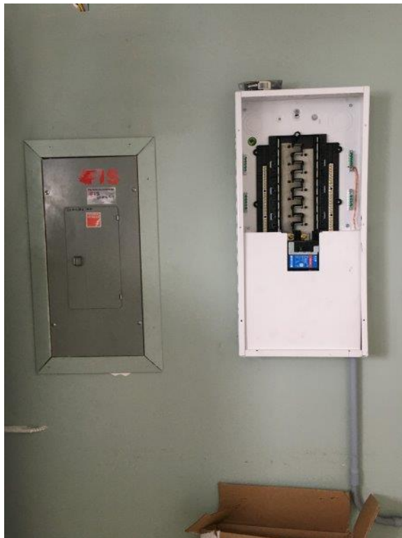
Photo 103 - New 200 A Panel Installed to Connect to Existing Hall Electrical Panel
