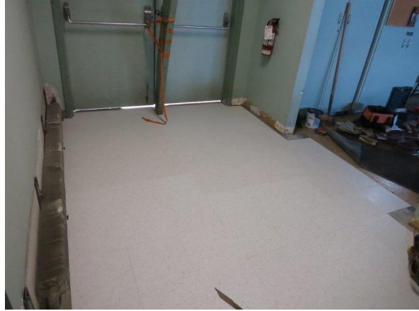
Photo 59 - New Floor Tile Being Installed at Front Entrance to Hall 2016
