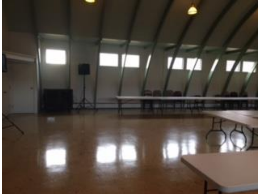
Photo 7 - Arch Rib Construction along the Straight Walls Intrude into Main Hall Space
