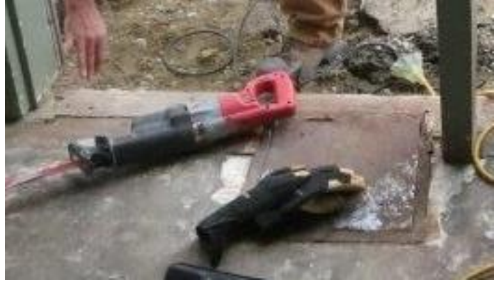
Photo 93 - Access Hatch under Entrance Floor with Door and Frame Removed
