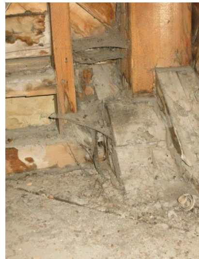
Photo 36 - Bell Tower Supported on Arch Rib
