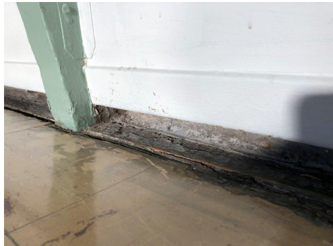
Photo 9 - Hall Interior Wall Showing Arch to Sill Plate Junction
