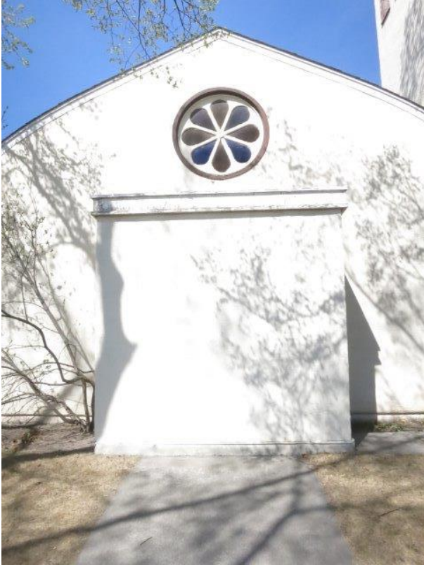
Photo 29 - South (Original Main) Entrance to Hall (Now Closed Off)
