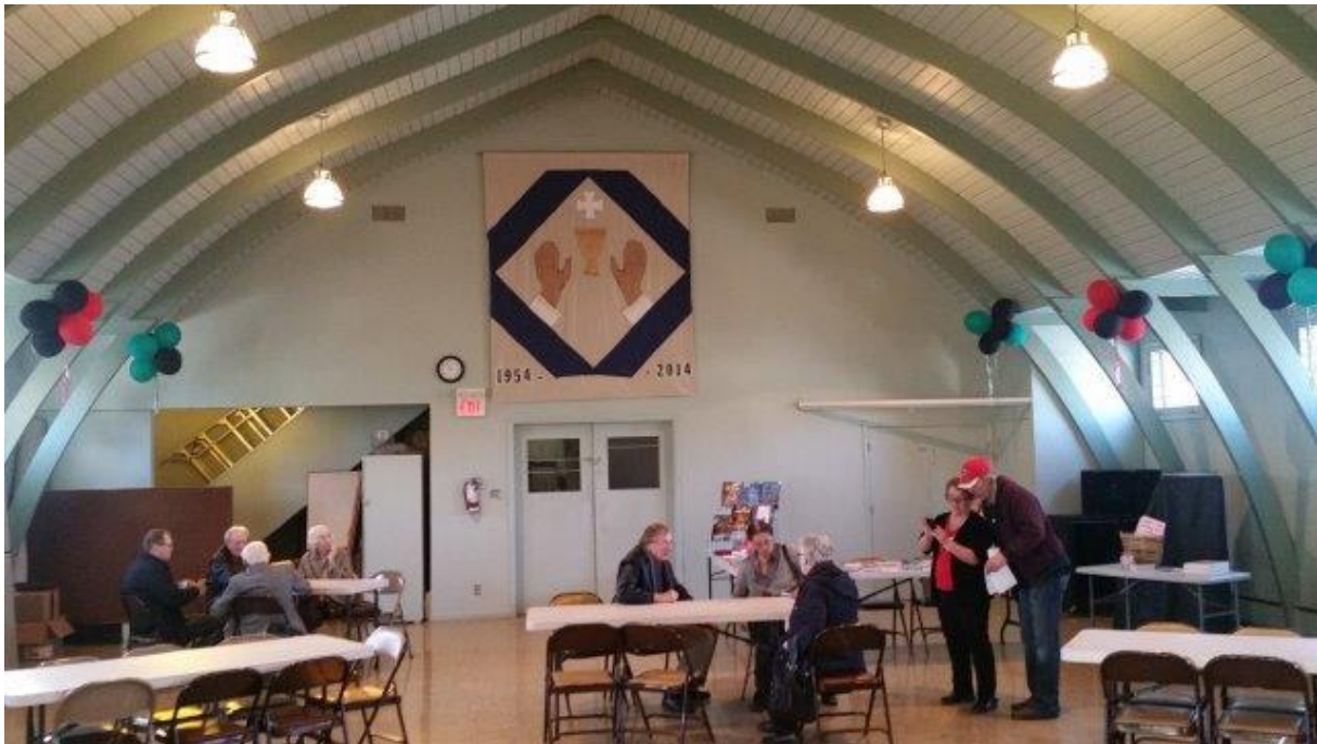
Photo 5 - Parish Hall South Wall (Original Entrance) in 2018
