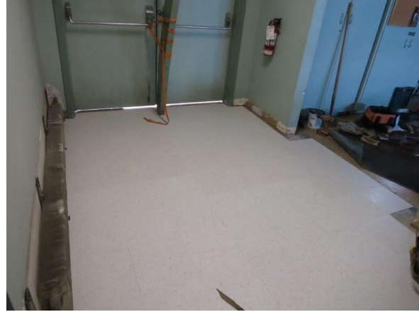
Photo 51 - New Floor Tile Being Installed at Front Entrance to Hall 2016
