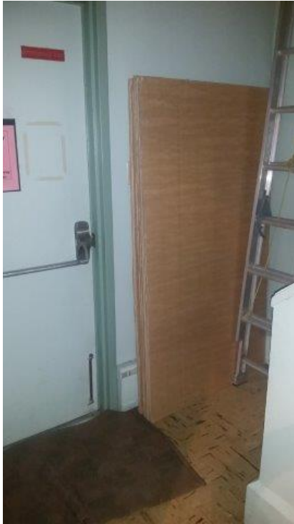
Photo 63 - Storage of Tall/Long Items at Stairway
