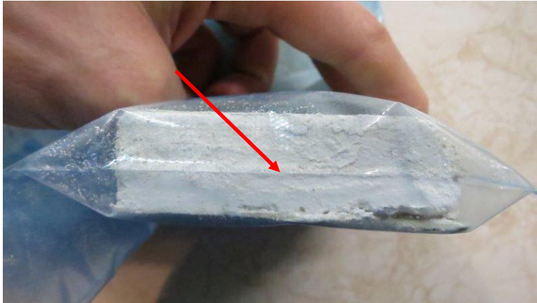
Photo 46 - Interior Wall Finish Material (drywall over hardboard)
