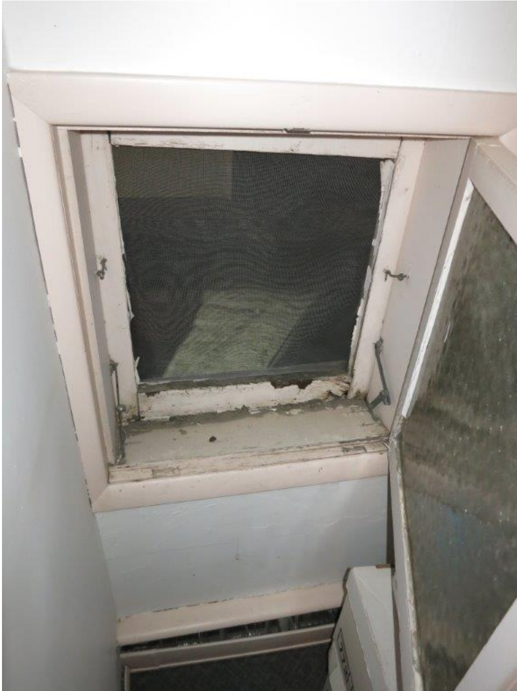
Photo 68 - Upper Office Original Window
