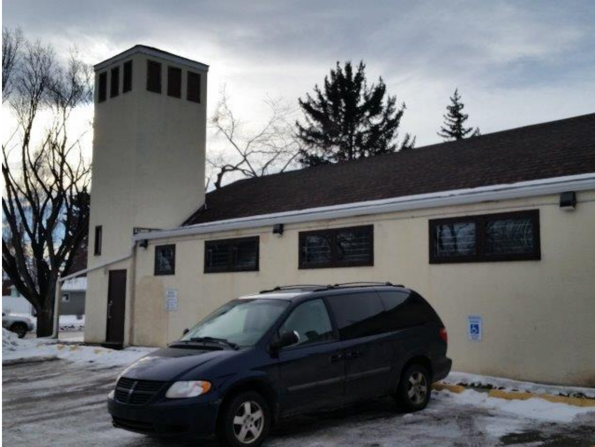
Photo 6 - East Exterior Side of Parish Hall ~2018
