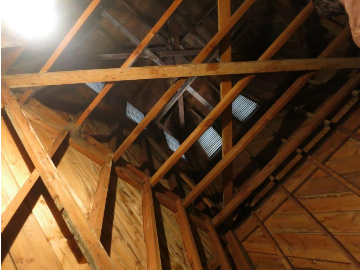
Photo 31 - Interior of Bell Tower
