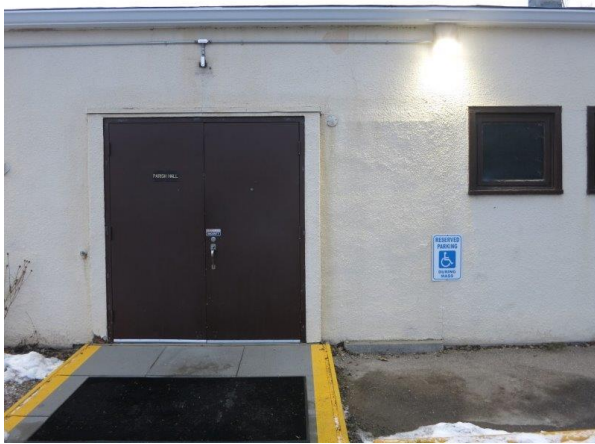
Photo 50 - Sloped Ramp added to Main Entrance 2016
