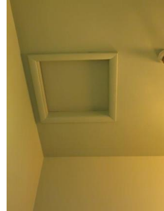
Photo 37 - Access Hatch to Bell Tower
