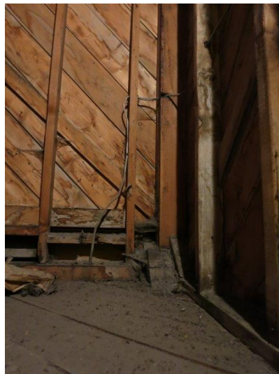
Photo 33 - Interior of Bell Tower Constructed on Top of Arch Rib
