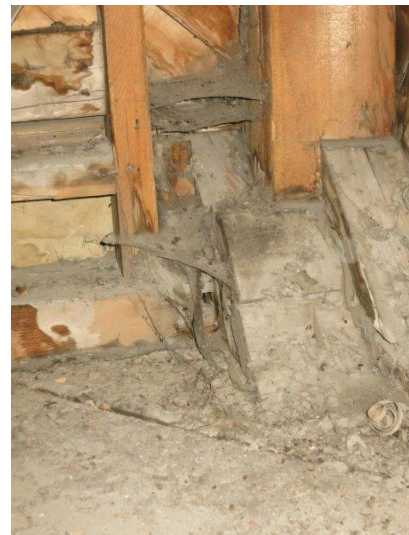
Photo 34 - Bell Tower Supported on Arch Rib
