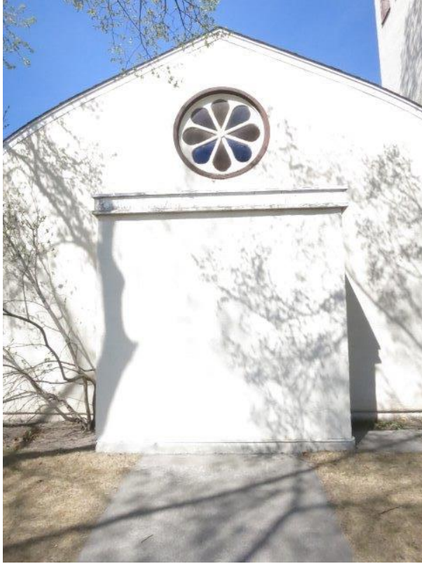
Photo 27 - South (Original Main) Entrance to Hall (Now Closed Off)
